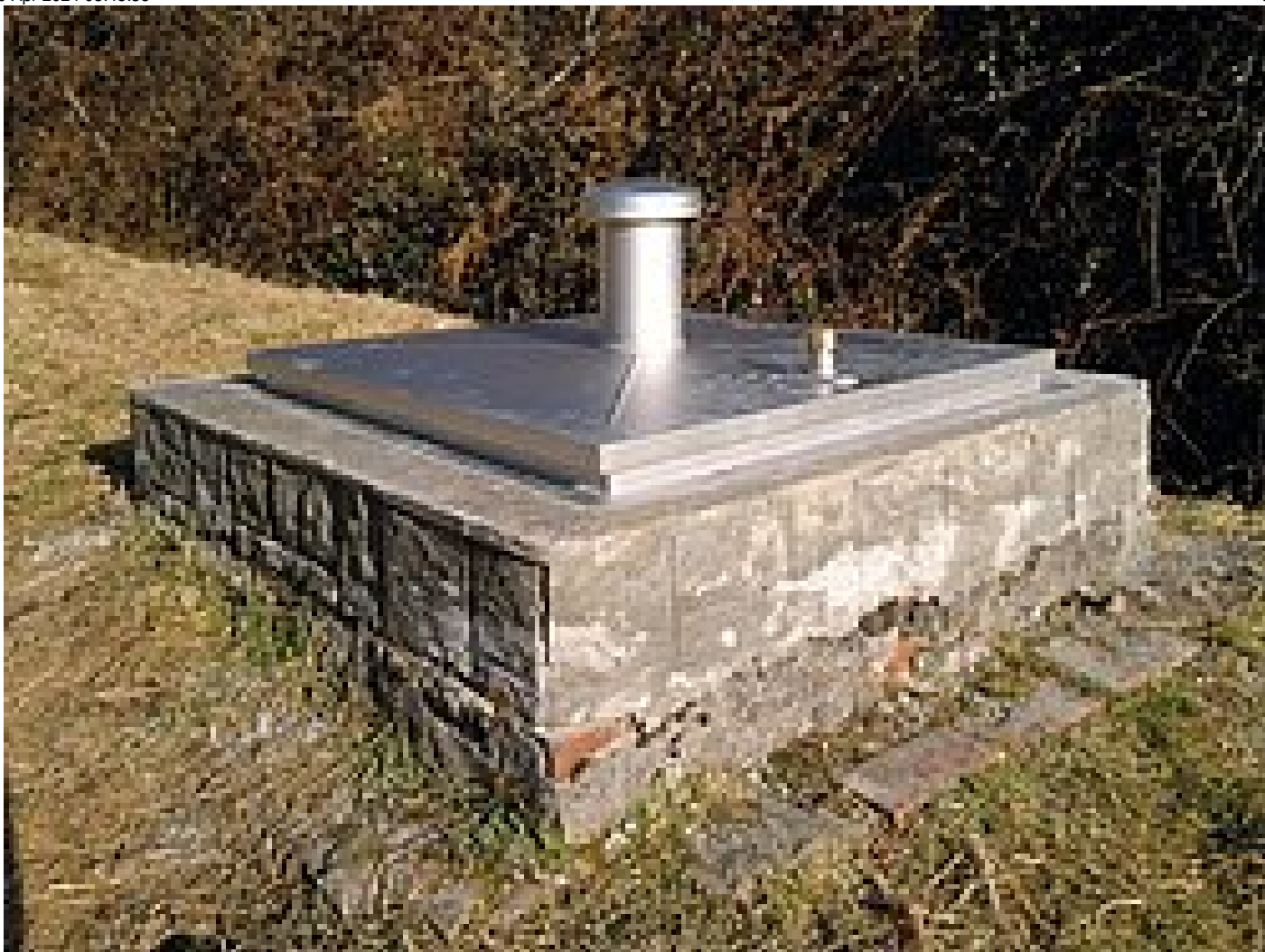
Weatherproof manhole cover
