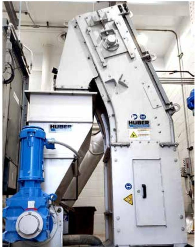
*The RakeMax® CF combines the benefits of maximum free screen surface and very high separation efficiency. Moreover, it is space-saving and reduces civil costs.*
