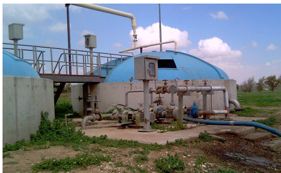
Static sludge thickener
